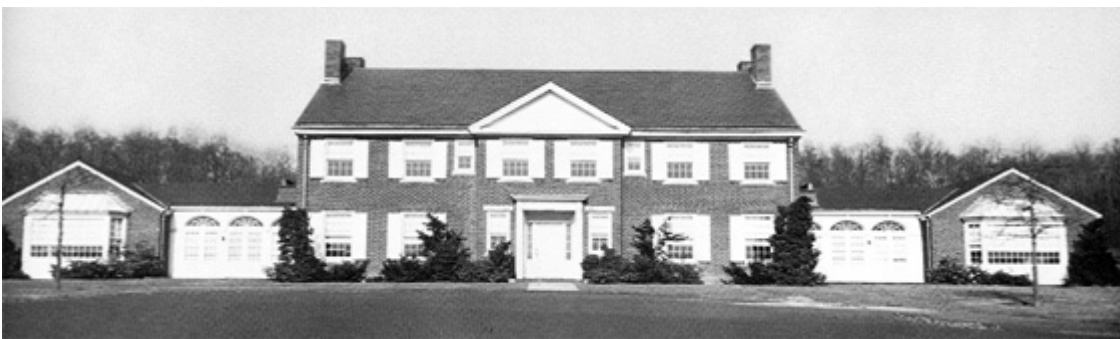
Buildings containing the dorms, dining area, kitchen, and nurses' station.
